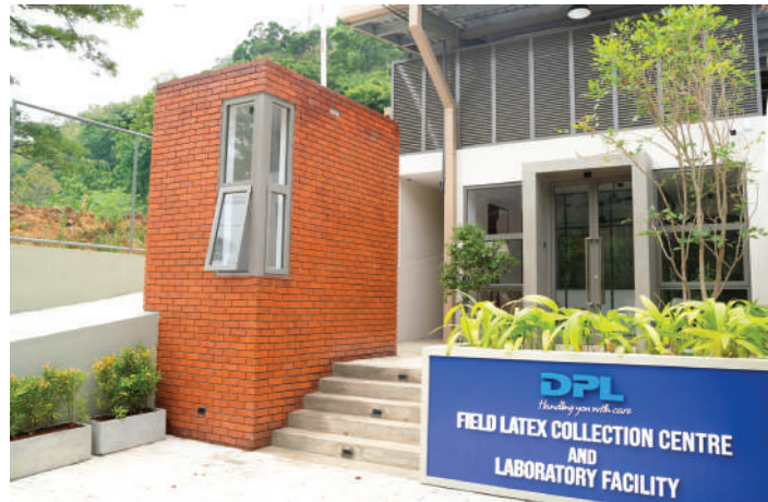
DPL Field Latex Collection Centre and Laboratory Facility.
